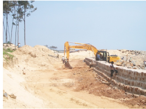
Fig. 6. Construction of sea dyke and eroded the dune bodies
