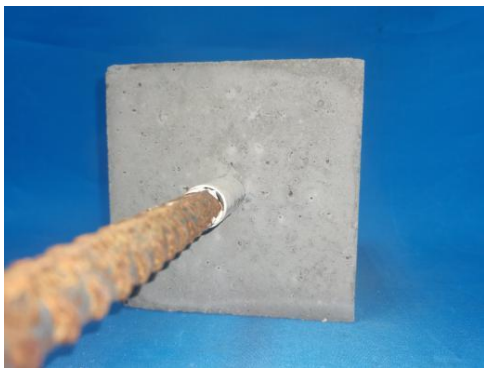
Fig. 2. Pull out damage
