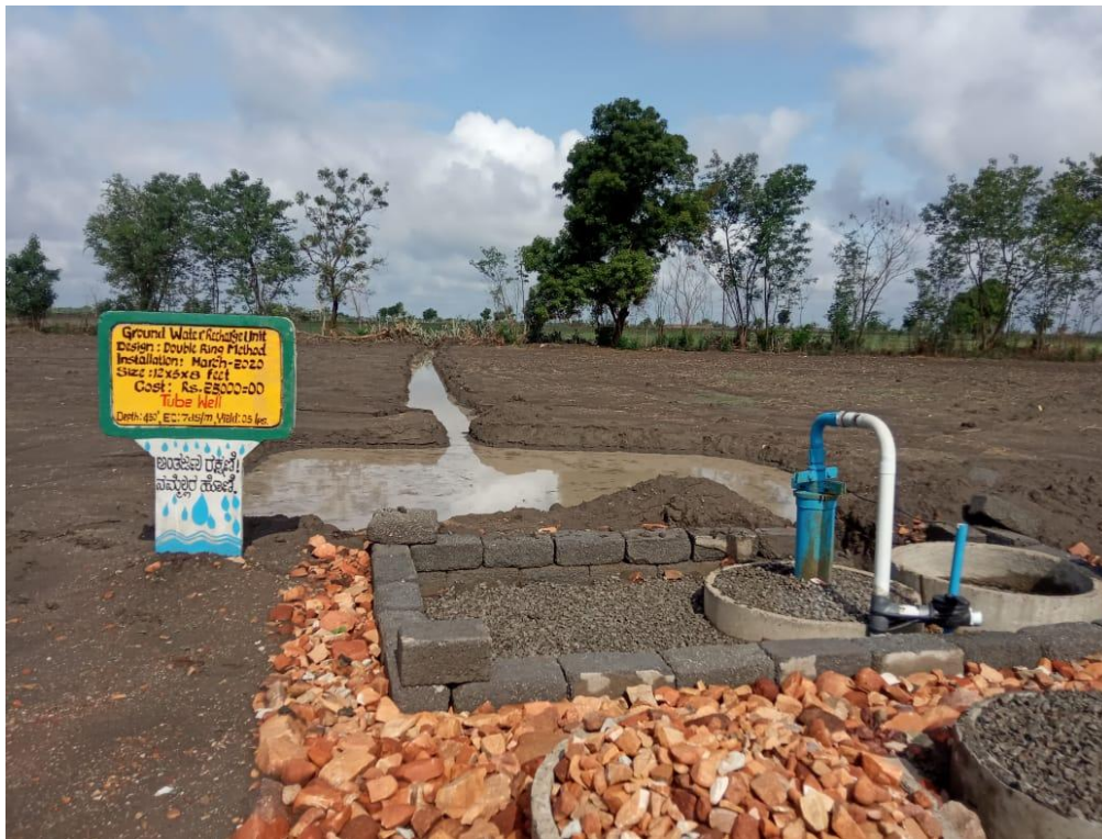
Fig. 2. A farm pond for tube well recharge at IWMRC Belavatagi (After recharging Rain fall events)
