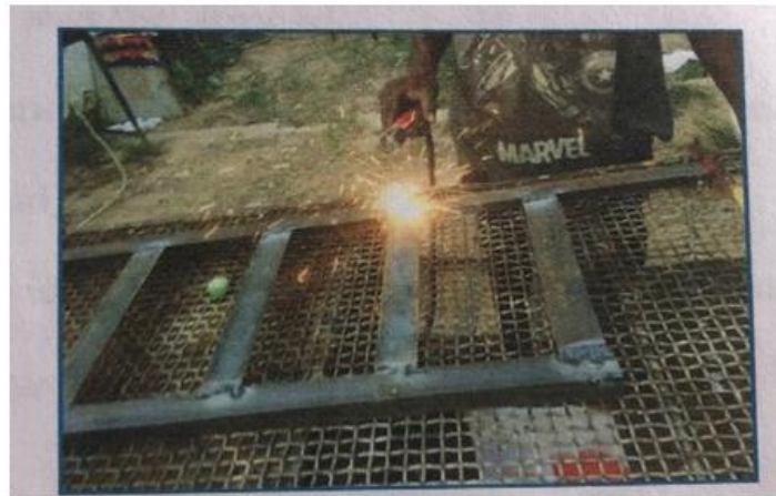
Fig. 12. Welding of the flat iron bar Source: Field work, 2021
