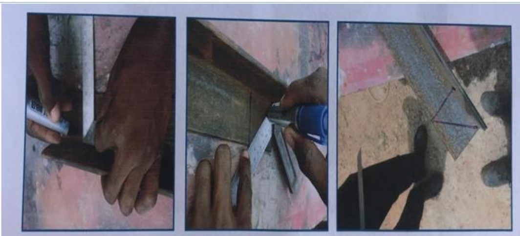
Fig. 10. Measuring of the iron bar Source: Field work, 2021
