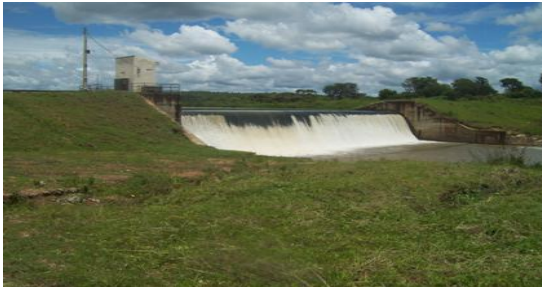
Fig. 1. Pictorial View of Unilorin Dam Source: [11]
