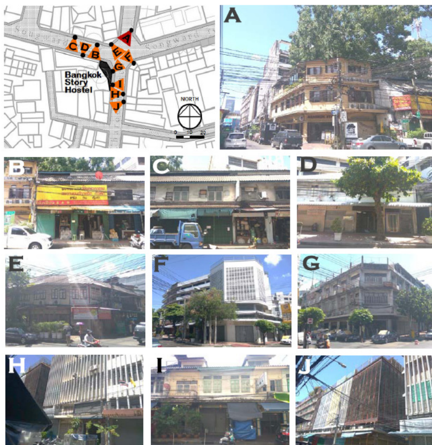
Figure 8. Survey map showing views of the surroundings and the building’s exterior
