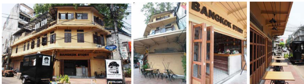
Figure 11. Views of the exterior, decoration, and timber accordion door on the ground floor
